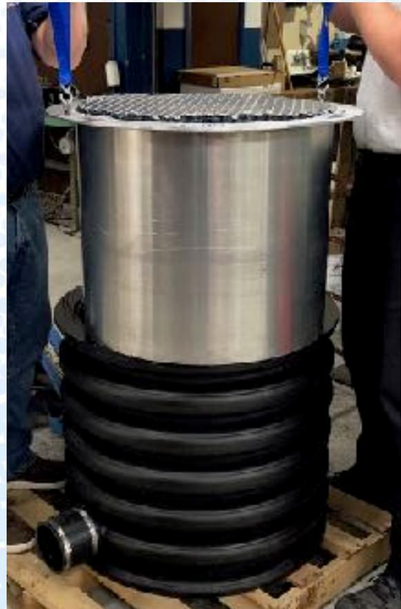
Next on the top of the aluminum Petro-Barrier Canister remove the Hex-head screws from flange, then using the Eye Bolts & lift the canister out of the corrugated housing and put with the Top Hat filter and replacement dirt filters for use after the HDPE housing has been installed.
