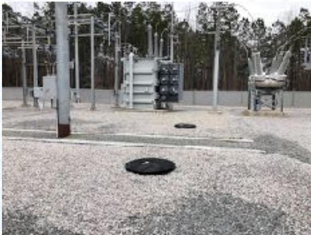
After the Petro-Barriers are installed they are accessed by removing the solid cover that is on the HDPE Gravel Guard. The gravel guards are backfilled with clean washed stone to limit as much dirt and debris as possible from getting into the Petro-Barrier dirt and debris filters.
