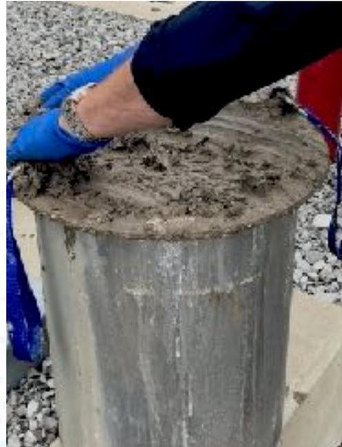
**X** This containment area was never cleaned before installing the Petro-Barrier Canister and instead of backfilling with clean washed stone dirty stone was used. Making the Petro-Barriers inoperable.
