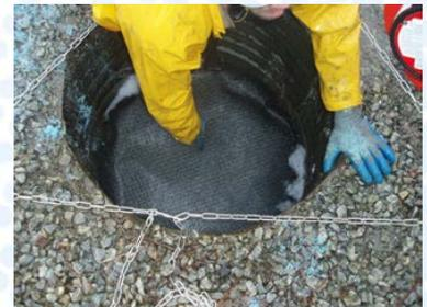
We go the extra mile. These **SPI Petro-Barriers™** were custom installed at a depth of 6'. Reinforced grating was bolted into the pipe and the **SPI Petro-Barrier™** Media was installed. This resolved an issue with the perforated pipe that had been previously installed.
