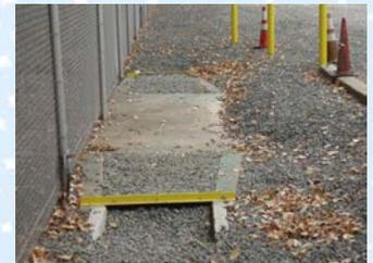
A Drainage trench 12" deep runs around the south side of this substation for water drainage. The trench leads to two (2) 30" wide x 5' long storm water drains. Grating is installed in the drains and crushed stone is used in the trench to slow the water flow. The SPI Petro-Barrier™ Media is installed and topped off with clean crushed stone. This system has been exposed to flooding since its installation with no drainage problems whatsoever.
