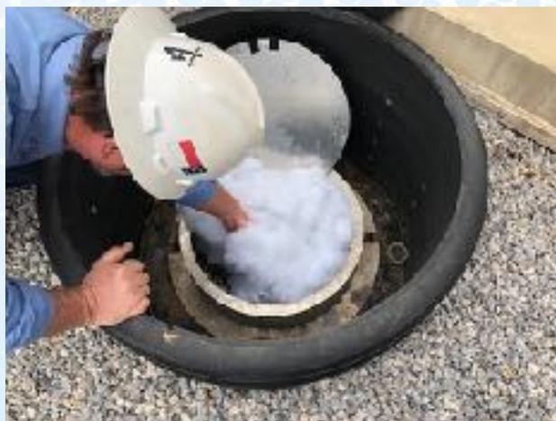
After a new installation the Petro-Barriers filters should be checked to ensure drainage after the first 1 - 2 months after install, this is when they will be the dirtiest.
