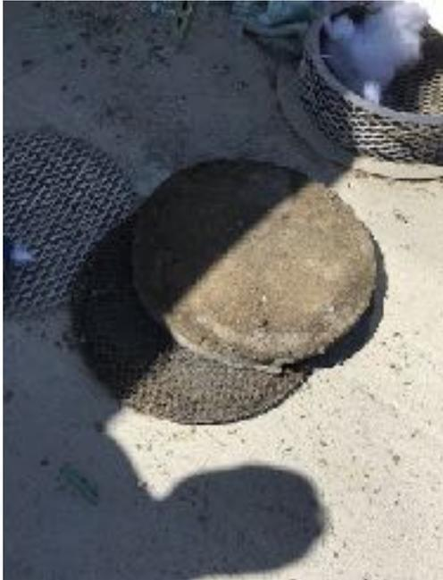
**X** This containment area drained well for 5 months and then slowed down. The dirt filters were never checked and changed causing the slow drainage.
